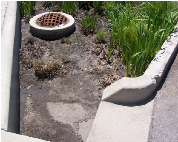
Sediment Accumulation
